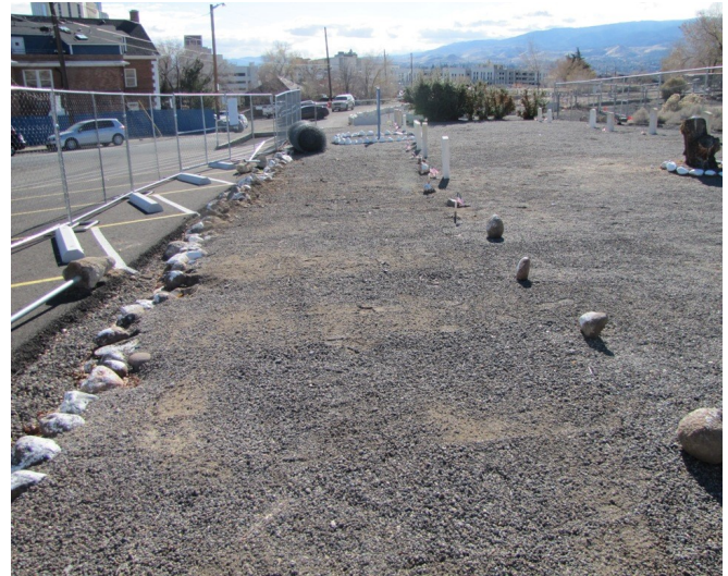
After Our Repair
