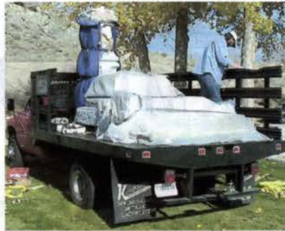
The GAR Civil War Monument returns in three sections - repaired, refurbished and ready for re-assembly !!
