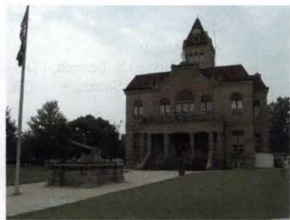
The above is the Greene County Courthouse in the City of Carrolton, Illinois. Next to the flagpole is a monument to all the soldiers and sailors who fought to preserve the Union during the Civil War donated by General William P. Carlin .
