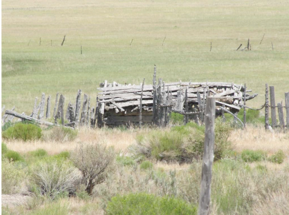
Remaining building looking east from road using telephoto lens.
